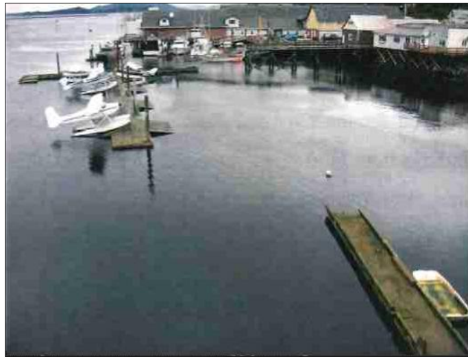
Figure 1: Existing Sitka SPB Looking North
