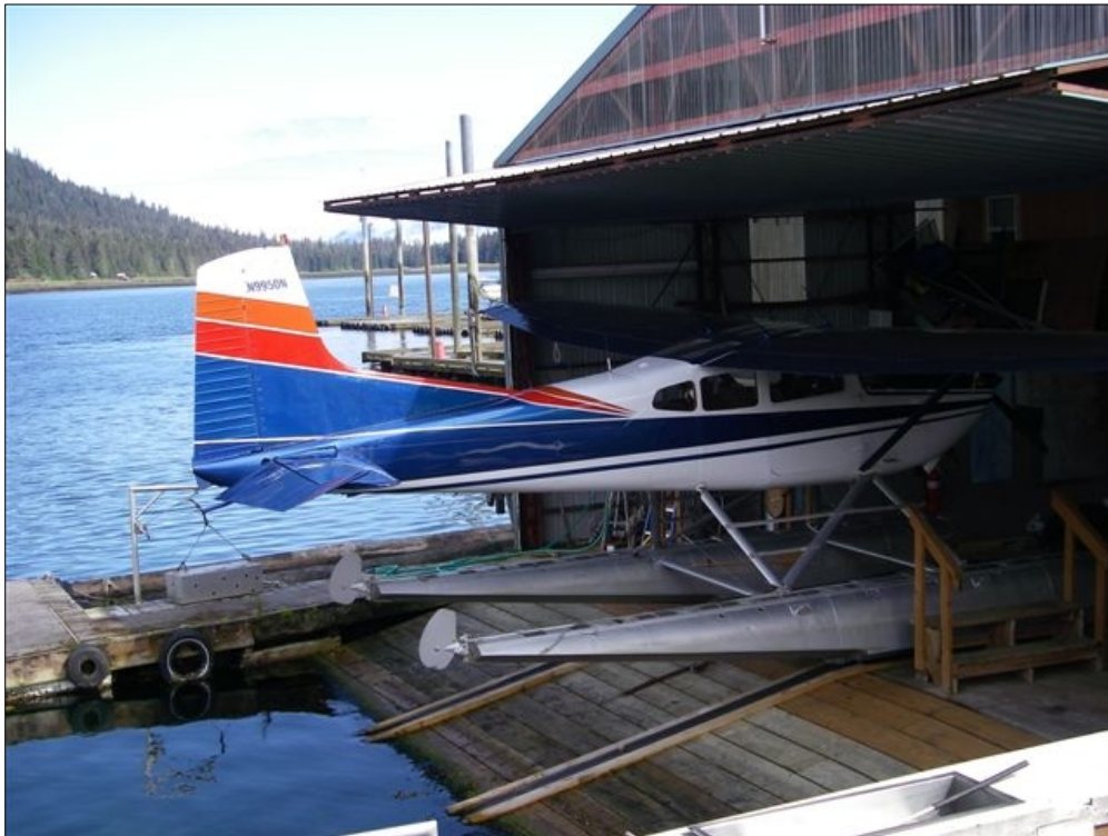
Figure 4: Floating Hangar - Petersburg
