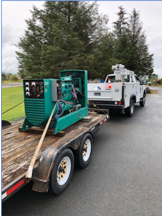
Old Generator on Trailer
