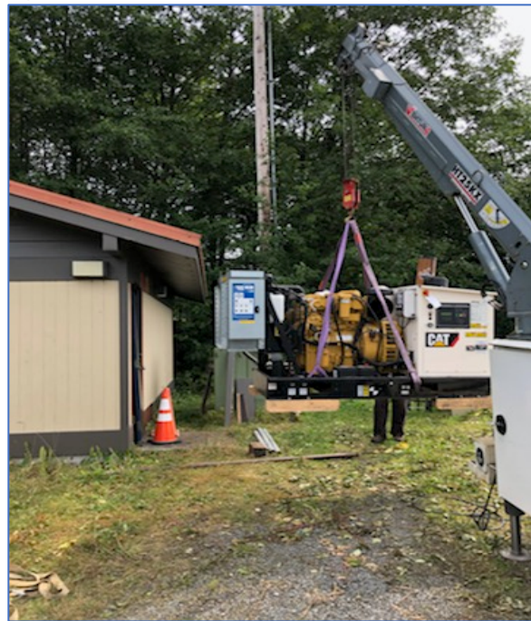
Hoisting the New Halibut Point Generator
